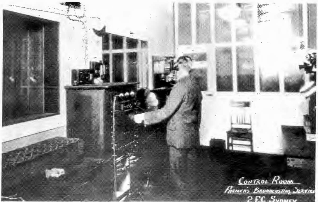
The earliest known photograph of an Australian radio broadcasting control room — 2FC's control room, which began service on December 5, 1923. It was built and equipped by AWA. (Courtesy AWA).
